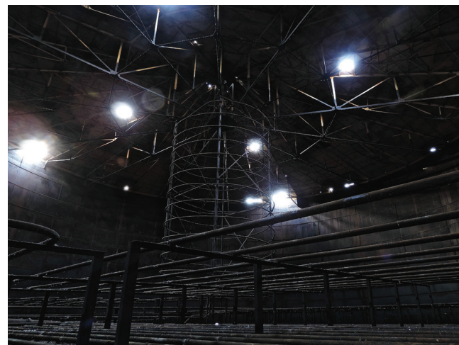
FIGURE 2. Oil tanks lack the visual features of Fig. 1, and require a new set of parameters to efficiently operate SLAM.
